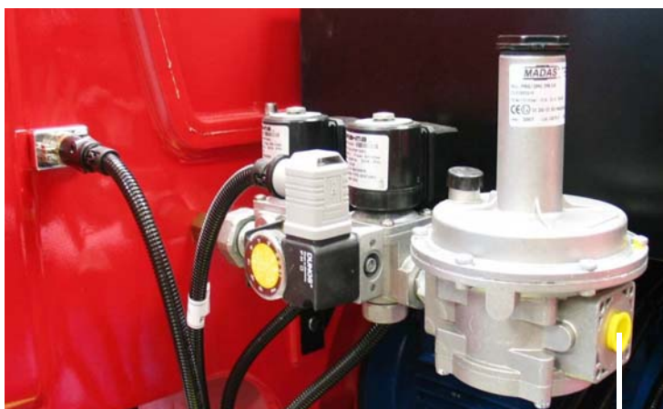
connection to the gas supply network - 1/2"
