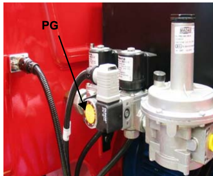
Fig. 27 - Gas pressure switch
