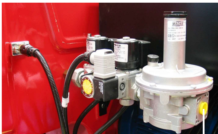
connection to the gas supply network - 1/2"
