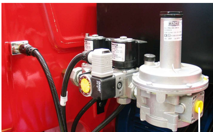
connection to the gas supply network - 1/2"
