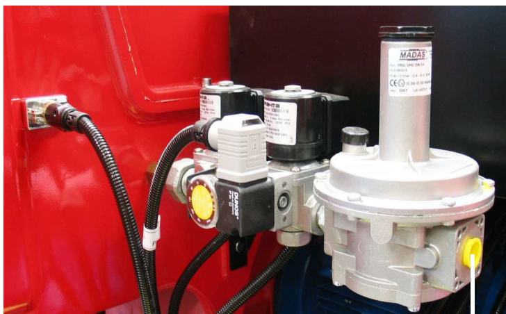
connection to the gas supply network - 1/2"
