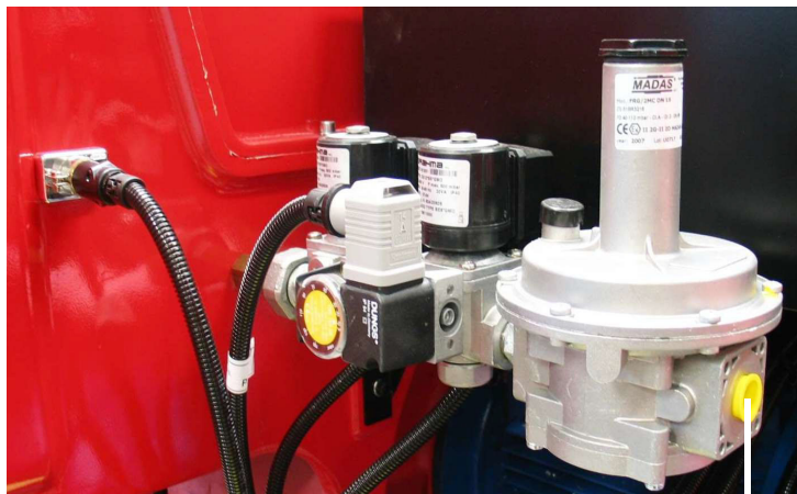
connection to the gas supply network - 1/2"
