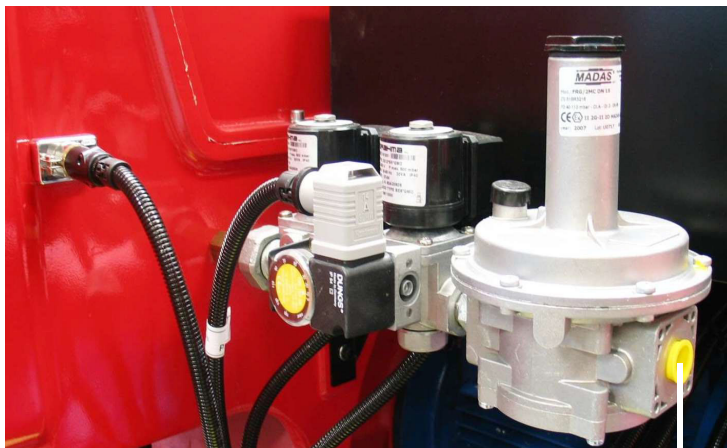
connection to the gas supply network - 1/2"
