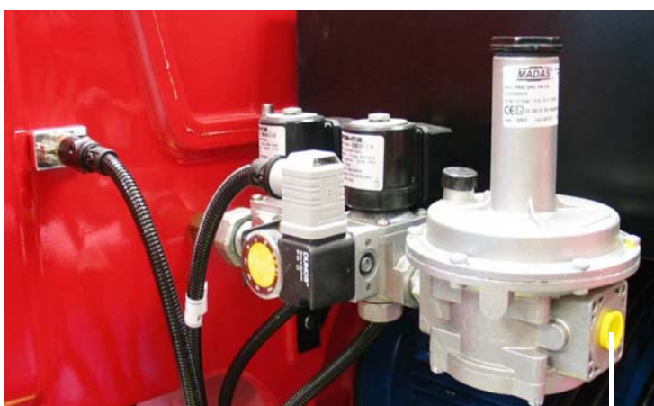
connection to the gas supply network 1/2"
