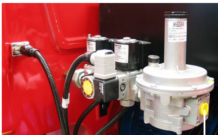
connection to the gas supply network - 1/2"
